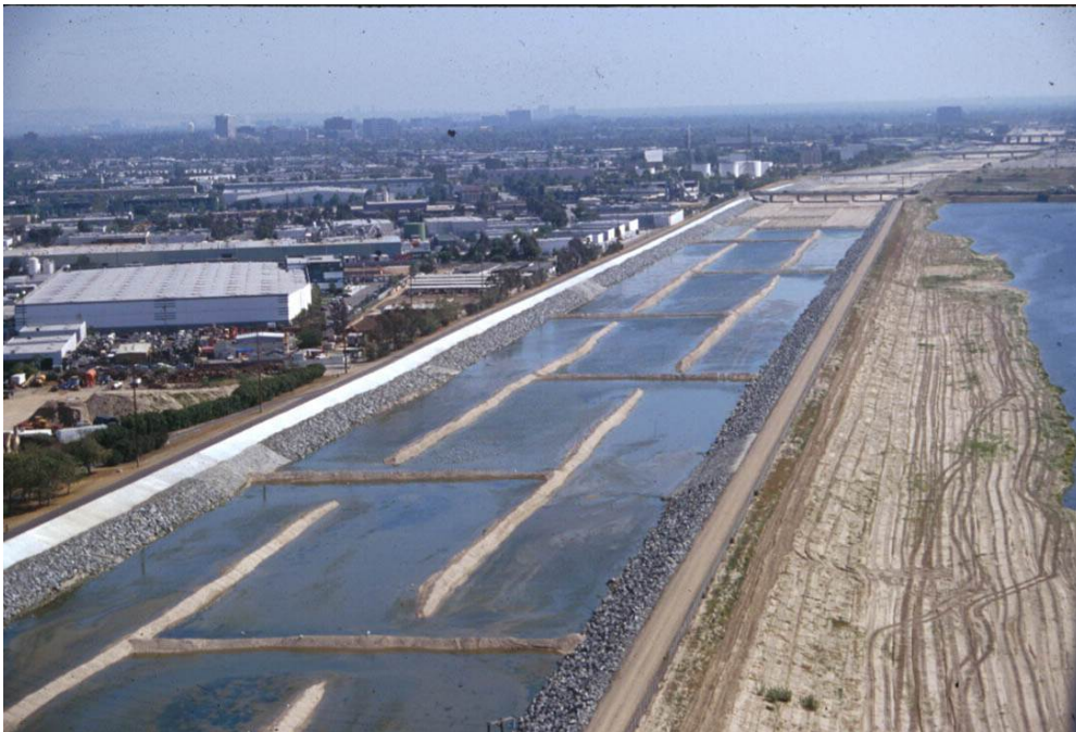
Figure 6-3 - "T" Levees in the Santa Ana River
